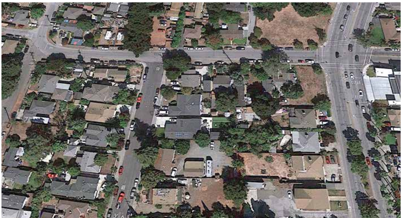
East Palo Alto. Imagery: Google Earth.
