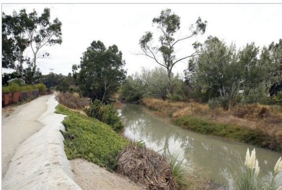
New levee built along the San Francisquito Creek.
