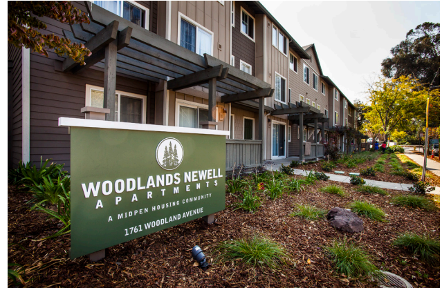
The renovated Woodlands Newell development, 49 affordable apartments for families in East Palo Alto.
