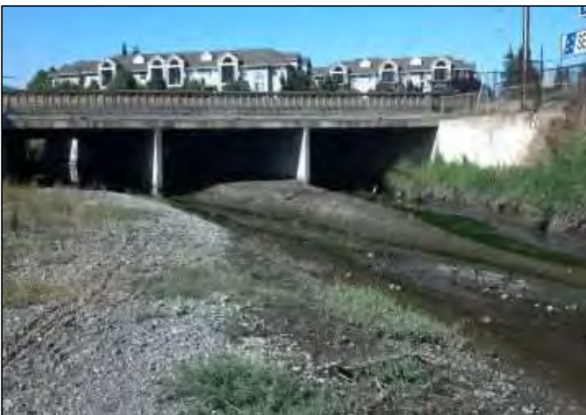
Photo 8. Highway 101 Bridge Over San Francisquito Creek
