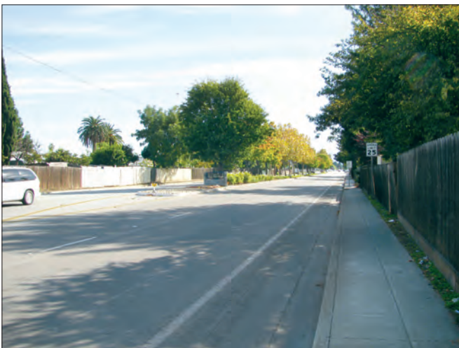
University Avenue streetscape with bike lane and narrow sidewalk.
