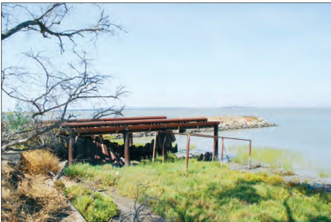
Former boat lift.
