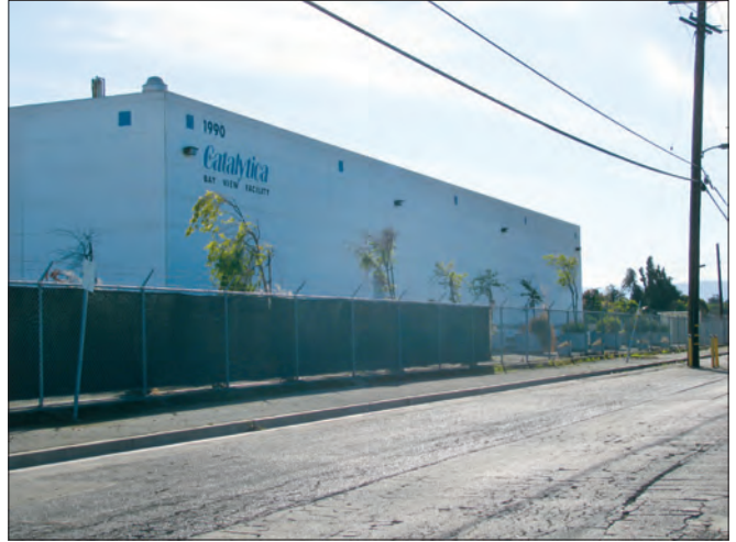
Former Rhône-Poulenc site at the east end of Bay Road.
