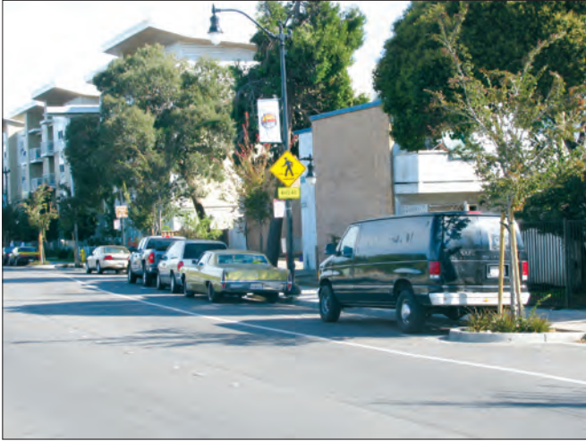
Recently built streetscape improvements and apartments near Fordham Street.
