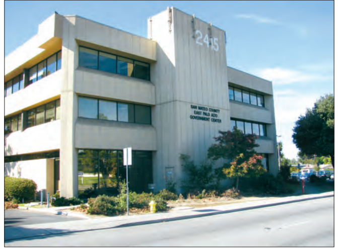
East Palo Alto City Hall.
