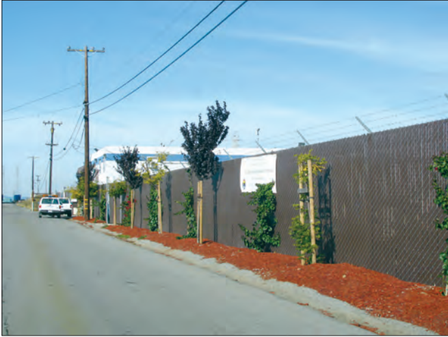
East Palo Alto Corporation Yard on Tara Street.
