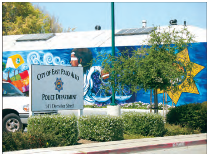
Police facility on Demeter Street.
