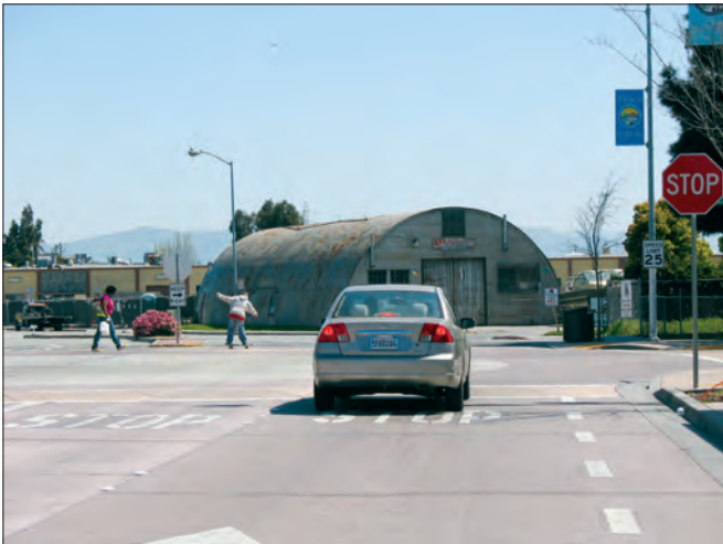
Quonset hut east of Bay Road/Clarke Avenue intersection.
