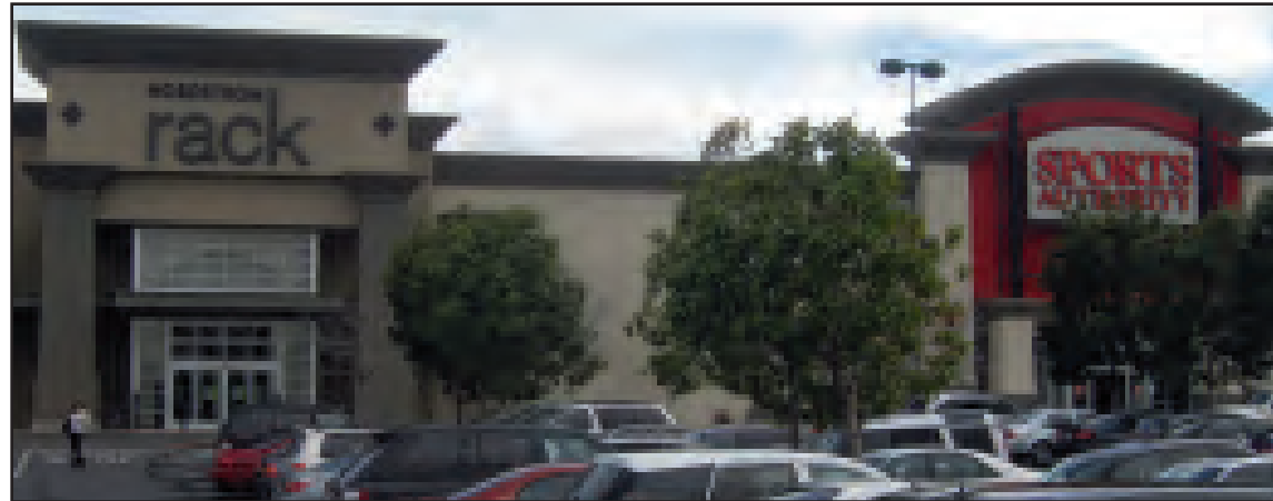
ENCOURAGED! Place signs above the front entrance of a commercial building ENCOURAGED! Design a sign to correspond with the size, height and shape of adjacent signs
