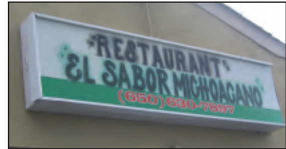
AVOID! Don't use internally illuminated cabinet signs.
