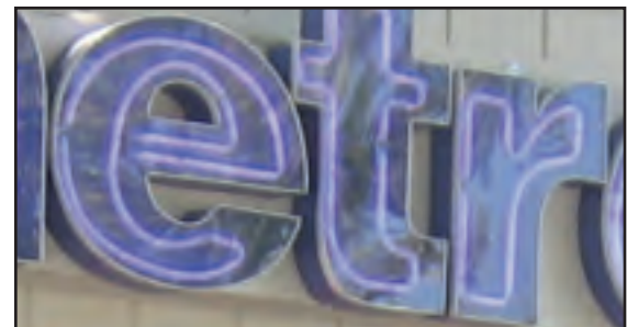
AVOID! Don't allow a sign's light source show (including bulbs and electrical equipment)
