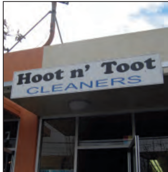
AVOID! Don't use signs that do not fit the wall space on the building
