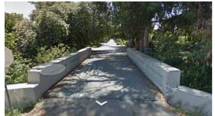
Existing Newell Bridge
