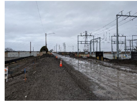
Bay Road Phase II Improvements
