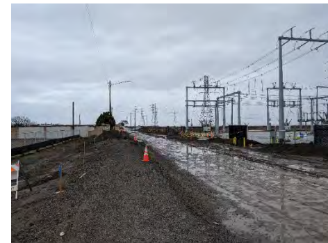
Bay Road Phase II Improvements
