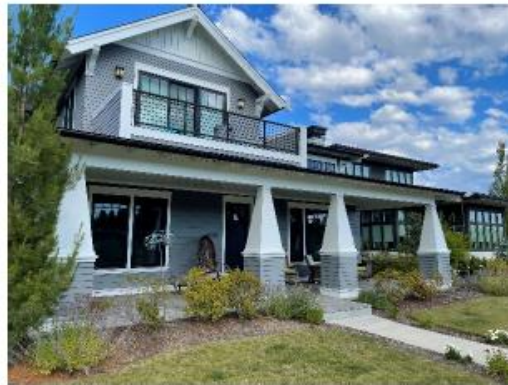
Balcony and covered front porch entry.
