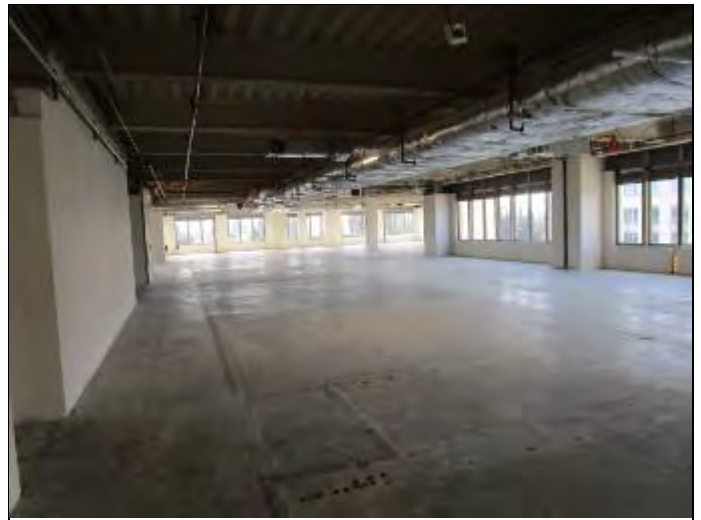
28. Vacant 5 th floor (1950 building)
