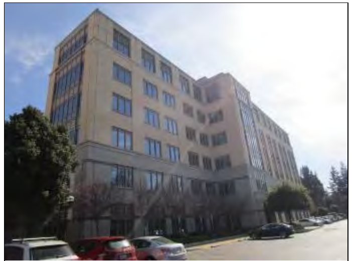
4. Northern and western sides of the 1900 University building
