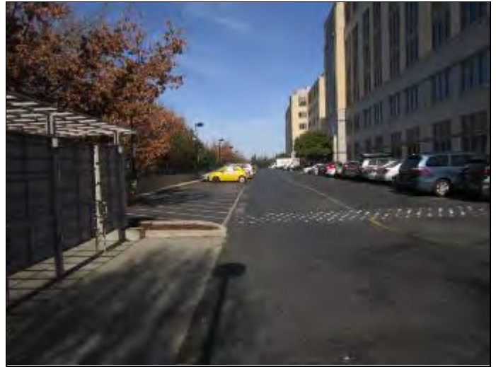
20. Asphalt-paved parking/drive area on the subject property
