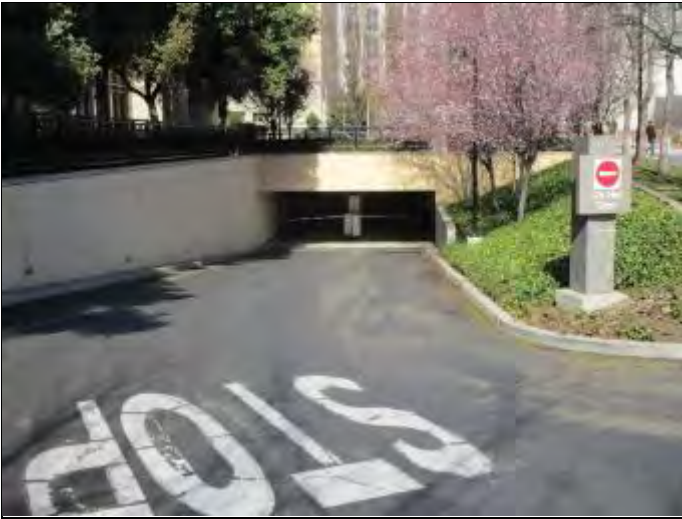
19. Underground parking garage exit
