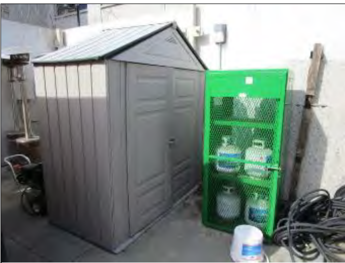
17. Propane cylinders and storage shed in the enclosure south of the 1950 building
