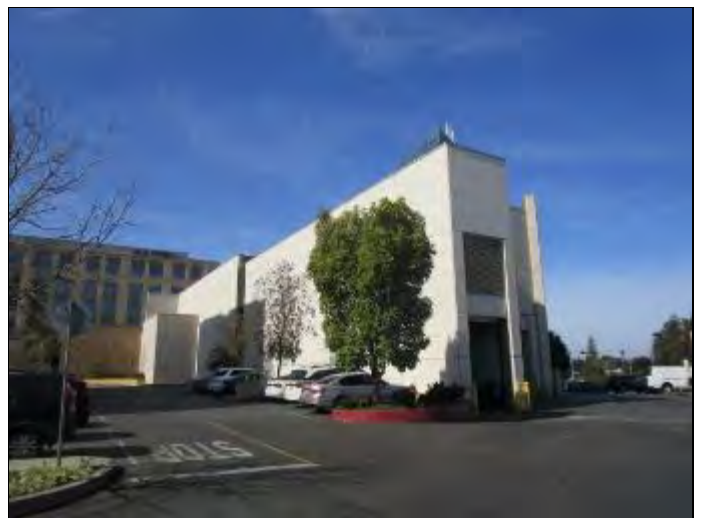
42. Four Seasons Hotel adjacent to the north
