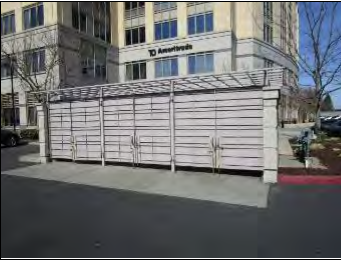
13. Dumpster enclosure south of the 1950 building
