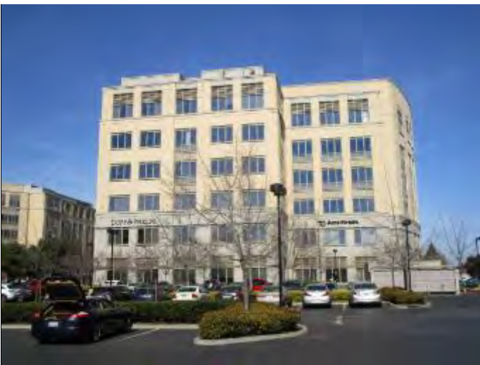
5. Eastern side of the 1950 University building
