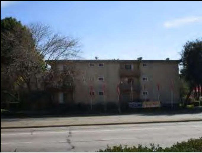
43. Apartment building adjacent to the east across East University Avenue
