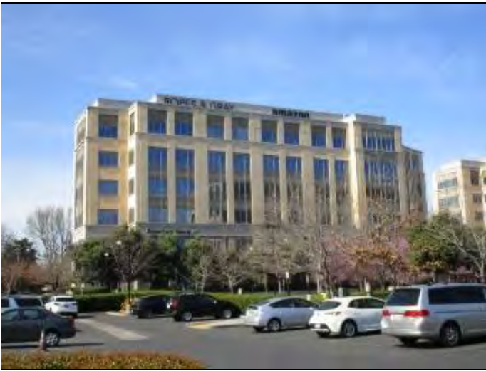
1. Eastern side of the 1900 University building
