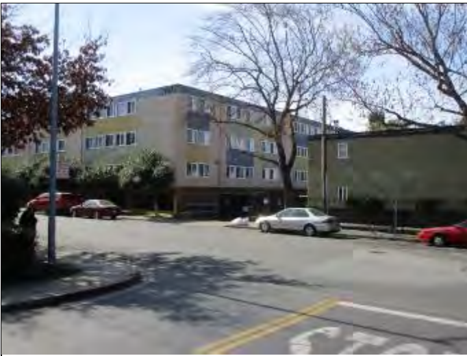
45. Apartment buildings adjacent to the west
