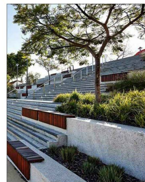
Terraced Walls and Stairs
