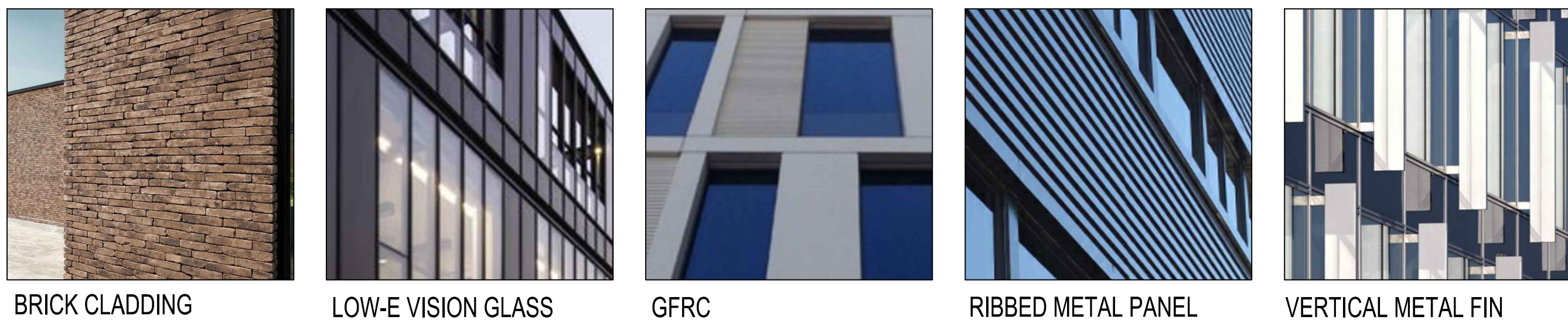
BRICK CLADDING LOW-E VISION GLASS GFRC RIBBED METAL PANEL VERTICAL METAL FIN
