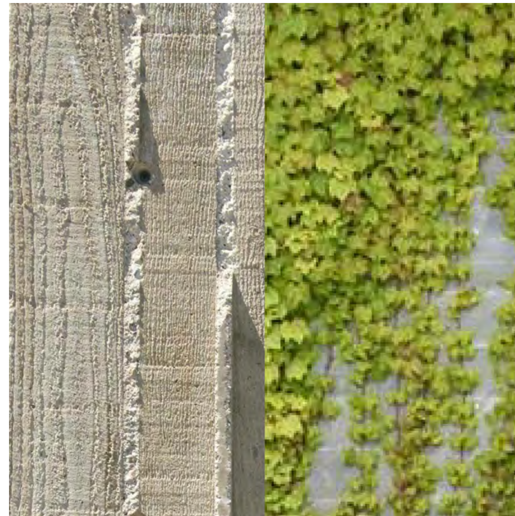
1 - Textured Concrete with Vine Cover
