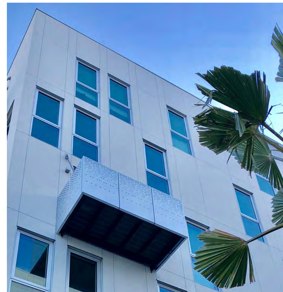
10 - Balconies with Perforated Metal Guardrails
