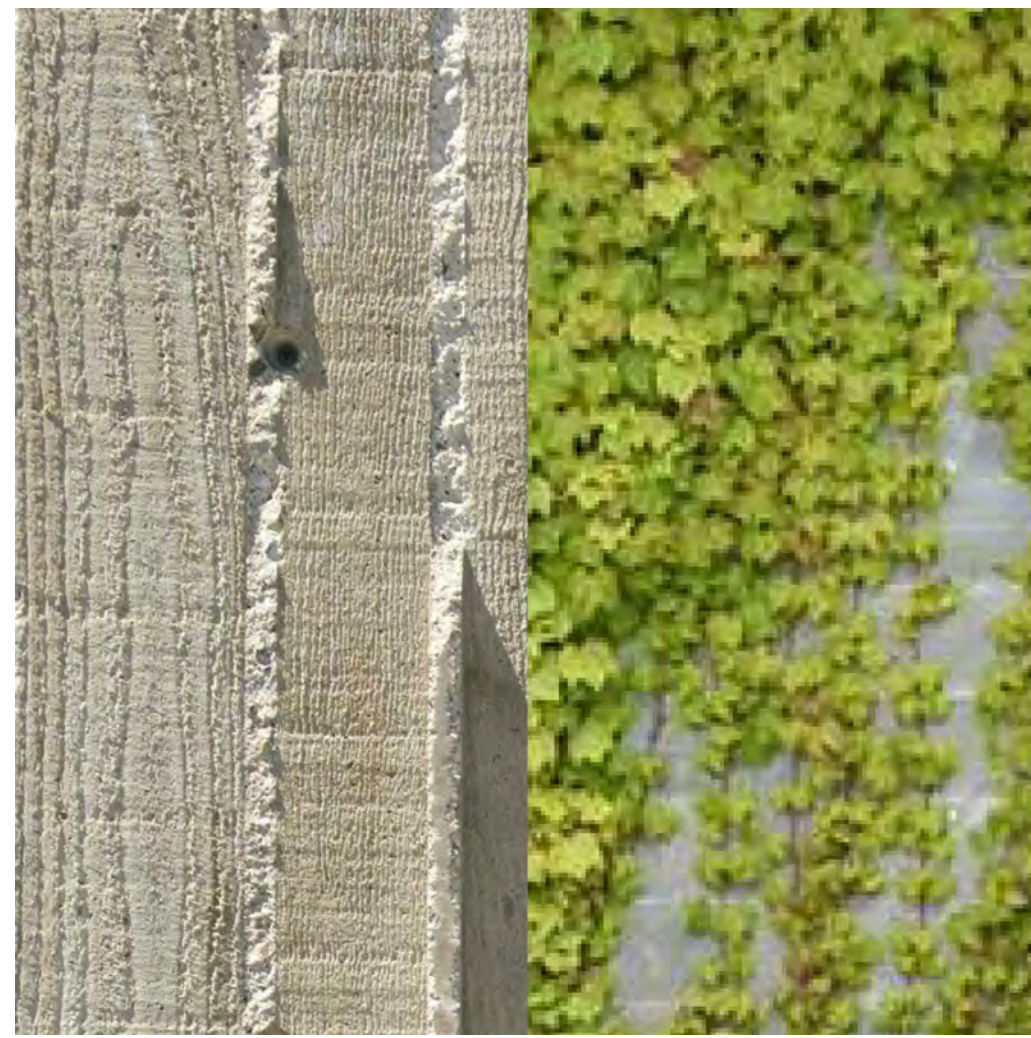
1 - Textured Concrete with Vine Cover
