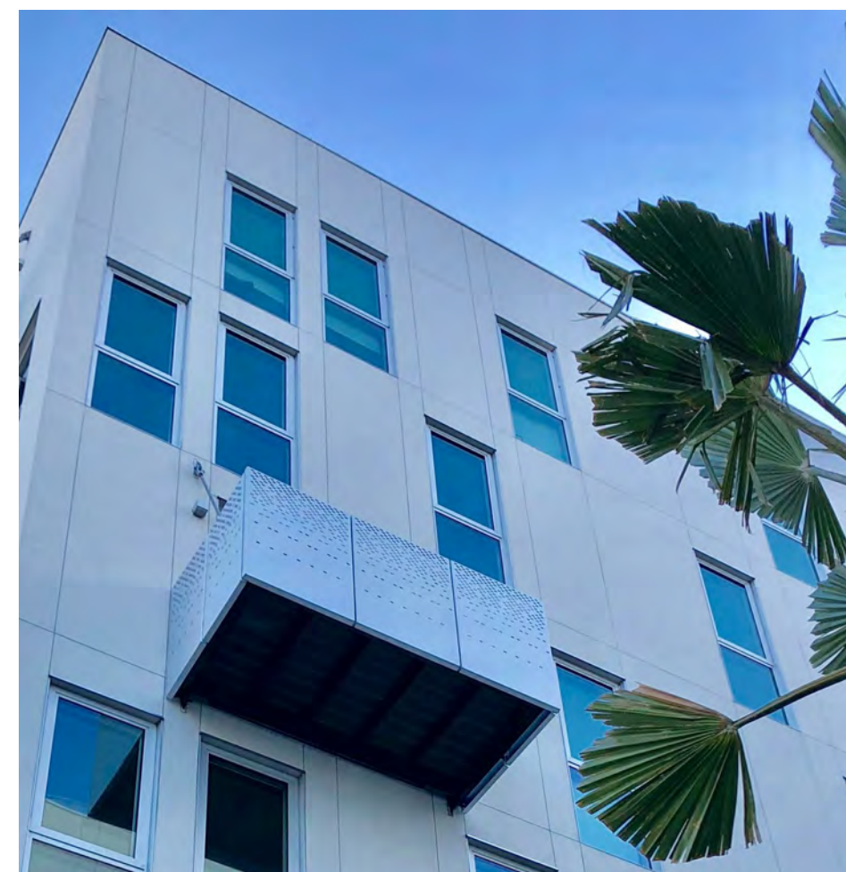
10 - Balconies with Perforated Metal Guardrails
