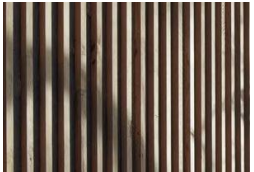
Stained Wood Plywood with 2x Vertical Wood Members
