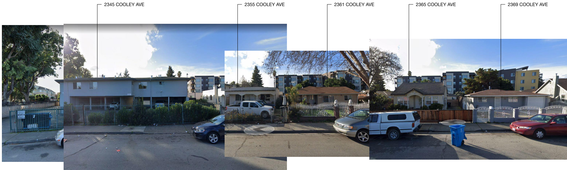
2 COOLEY AVE WEST ELEVATION
