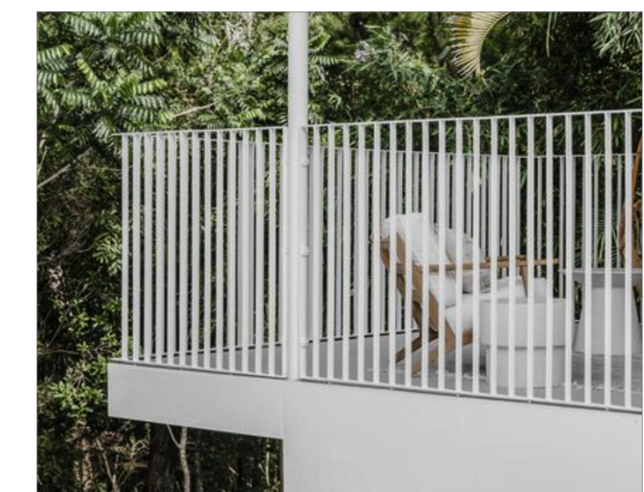
GALVANIZED STEEL GUARDRAIL PRIMED AND PAINTED WHITE
