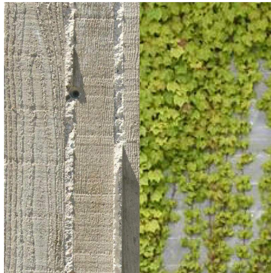
1 - Textured Concrete with Vine Cover
