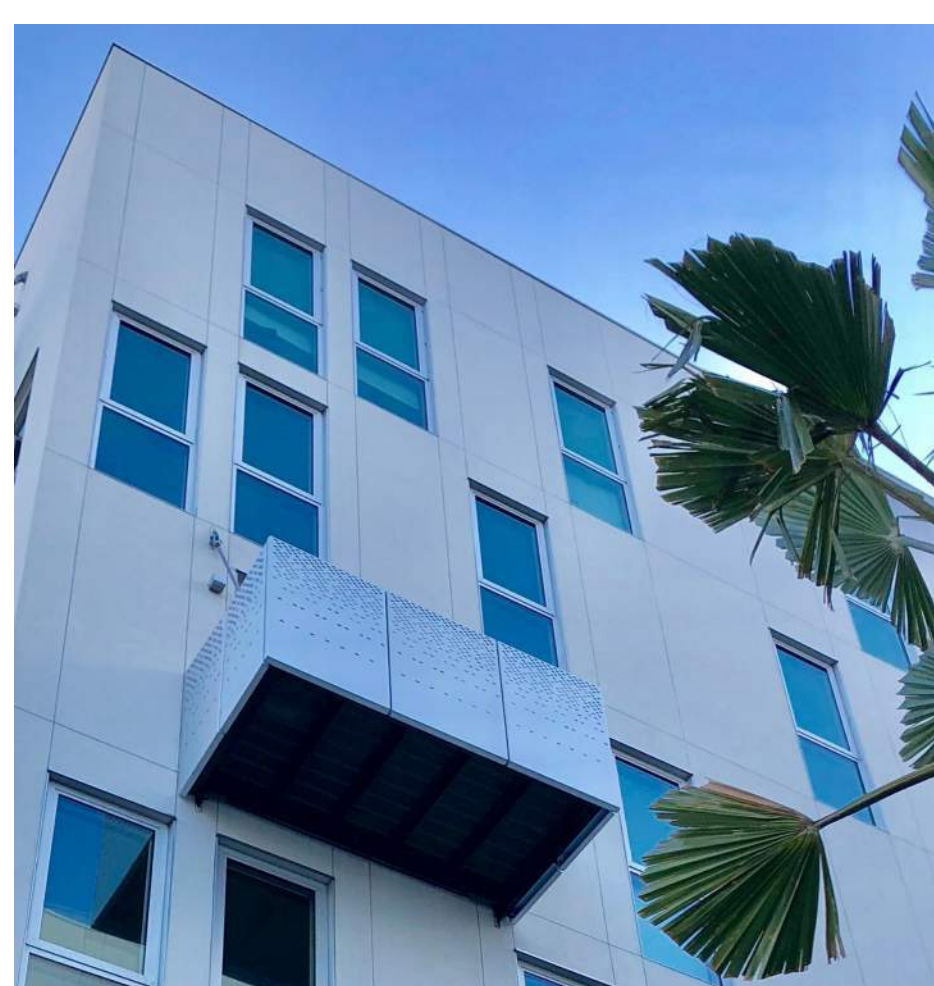
10 - Balconies with Perforated Metal Guardrails
