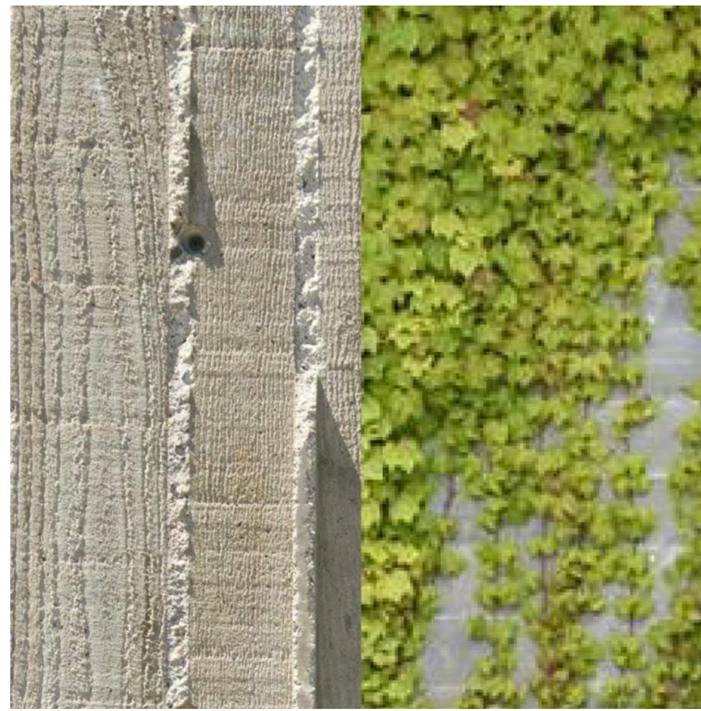
1 - Textured Concrete with Vine Cover
