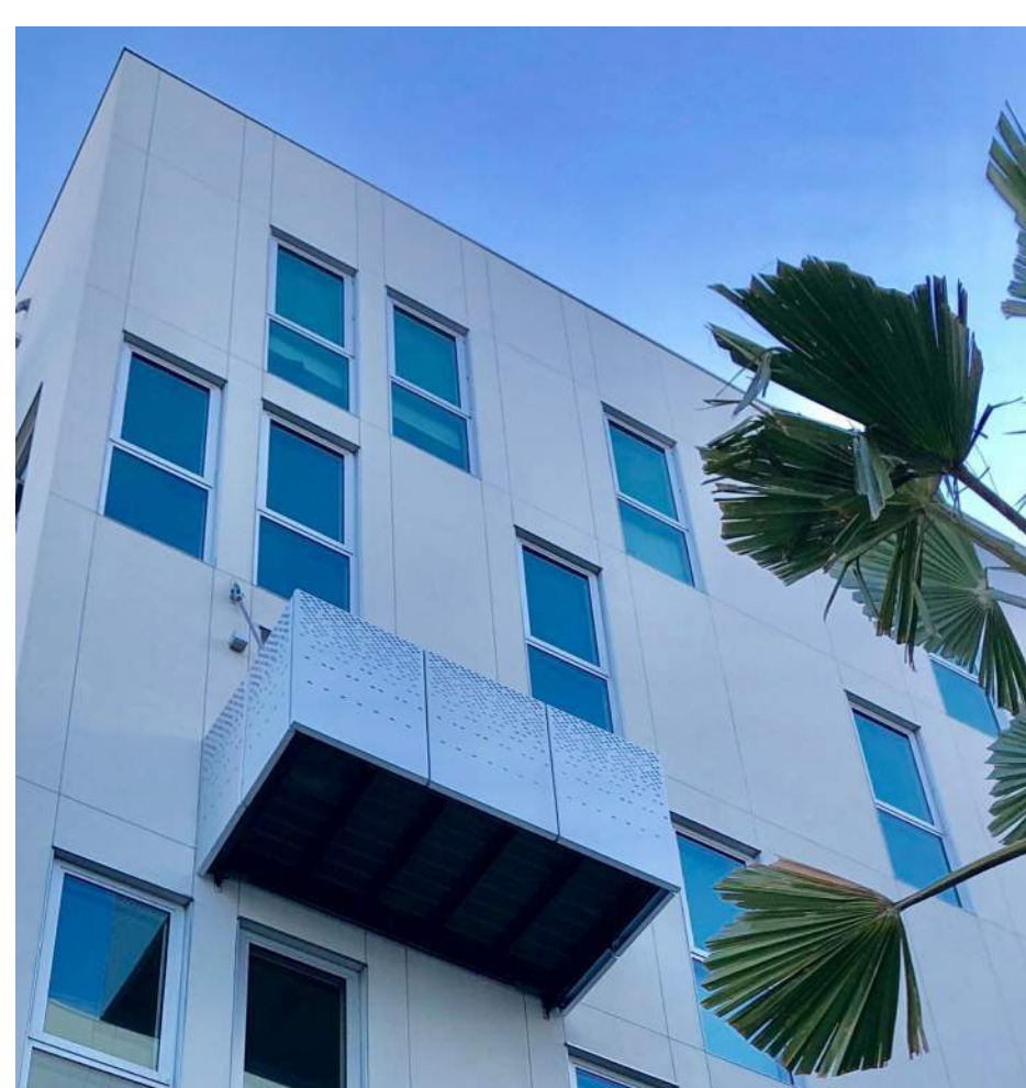
10 - Balconies with Perforated Metal Guardrails
