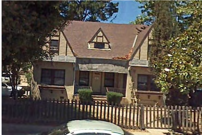
Figure 15. 2043 Euclid Avenue in July 2007. Source: Google Street View.
