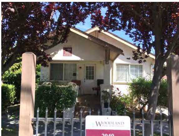
Figure 6. Main residence at 2040 Euclid Avenue, looking east.
