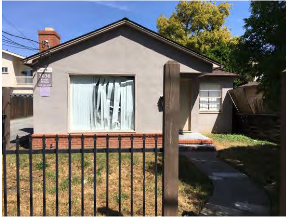
Figure 4. Main residence at 2036 Euclid Avenue, looking east.
