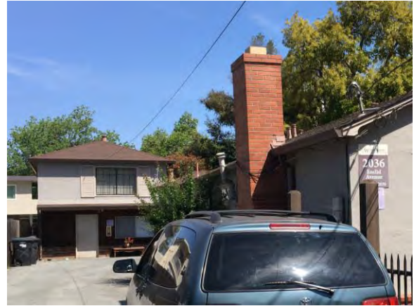
Figure 5. Detached two-story secondary residential building at the rear of the 2036 Euclid Avenue property, looking east.
