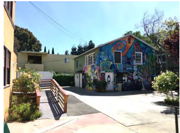
Figure 10. 420 E. Okeefe Street, the property west of 2043 Euclid Avenue, looking south.
