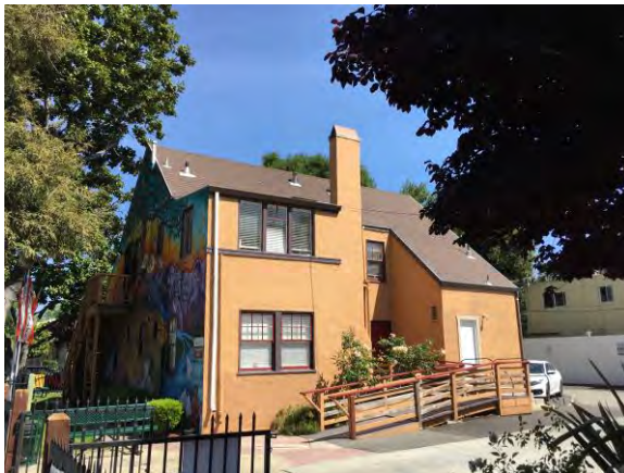
Figure 9. Rear of 2043 Euclid Avenue, looking southeast.
