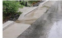
NEW CURB & GUTTER
