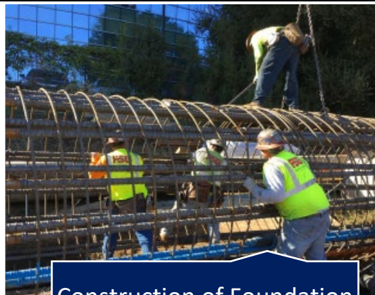
Construction of Foundation Reinforcement
