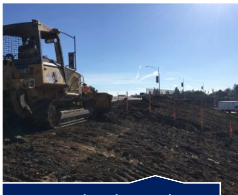
Finished Grade along Embankment
