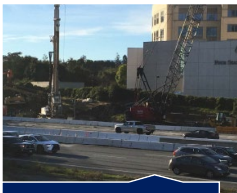
View of Structural Excavation
