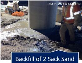
Backfill of 2 Sack Sand Slurry for Hole Caving
