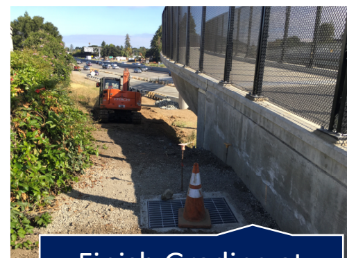
Finish Grading at Abutment 5
