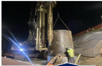
Permanent Steel Casing Being Placed
