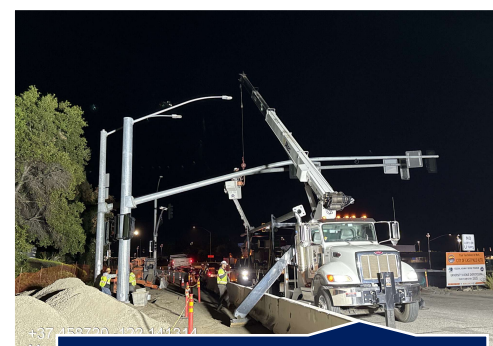
Traffic Signal Switch- Over
