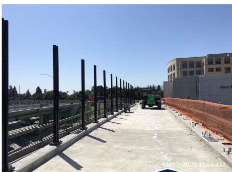
Bridge Railing Installation
