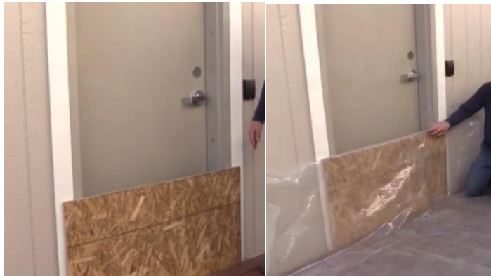
Image 2 & 3: Placement of plywood and plastic sheet
