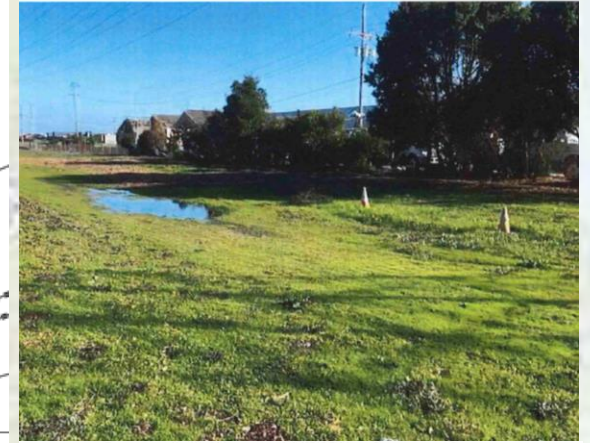
Storm Drain Discharge Outfalls in Private Property at Stevens
