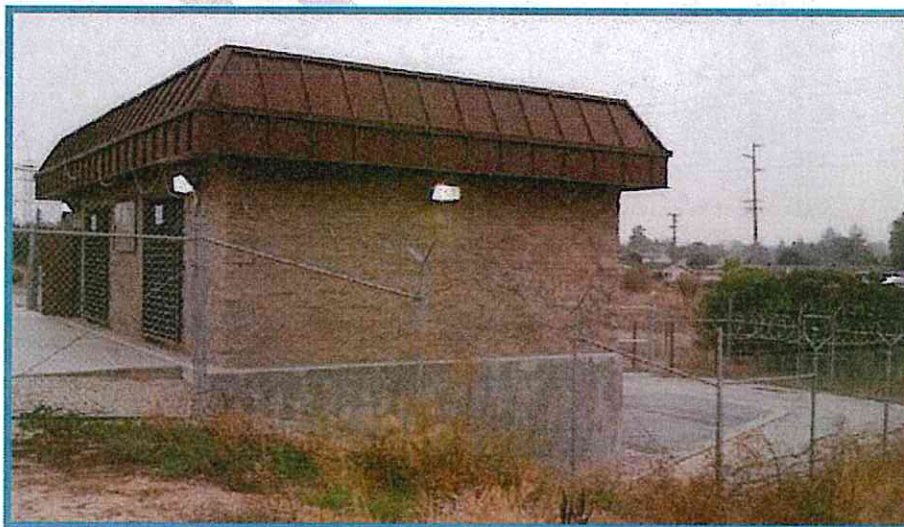
Figure 4-5: O'Connor Pump Station
