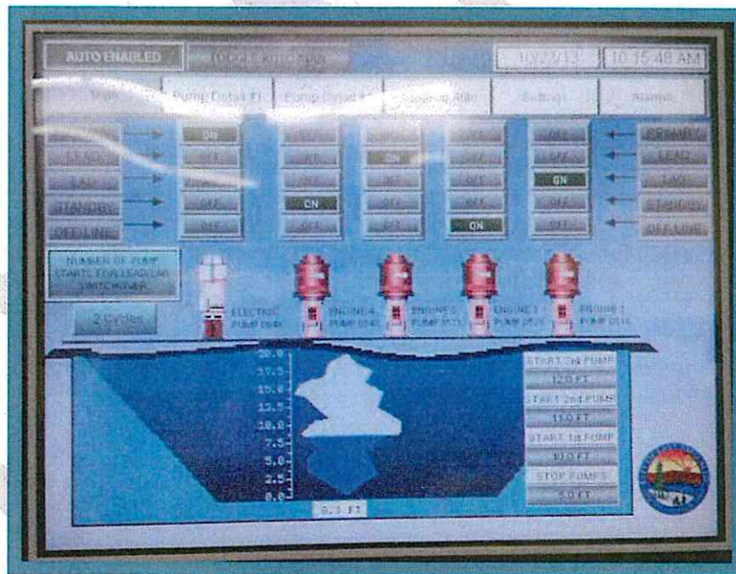
Figure 4-6: PLC Control Screen
