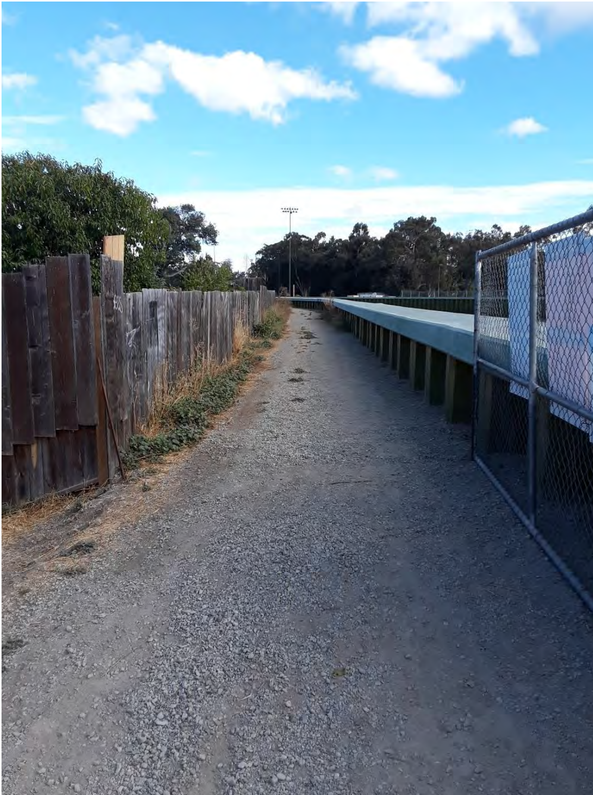
Figure 40 SFCJPA Flood Protection and Trail Resurfacing Project
