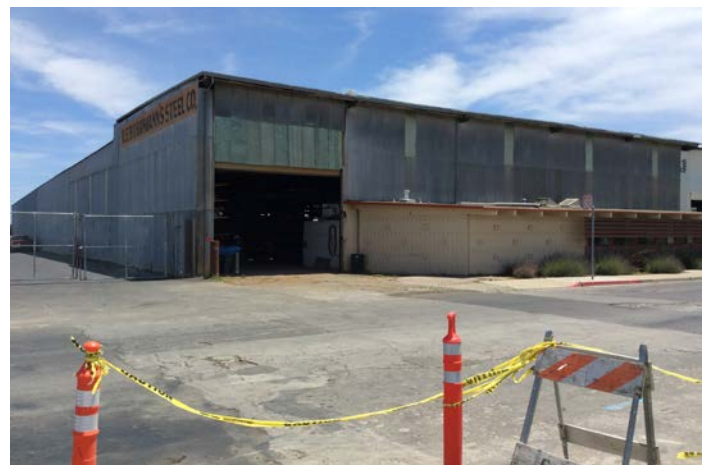
Photo 18: View of property immediately south of the site.
