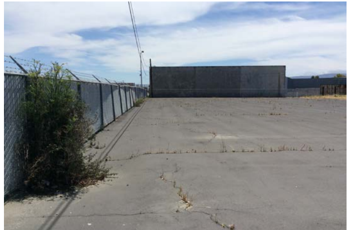
Photo 4: View of asphalt cap located along northeast side of the site.
