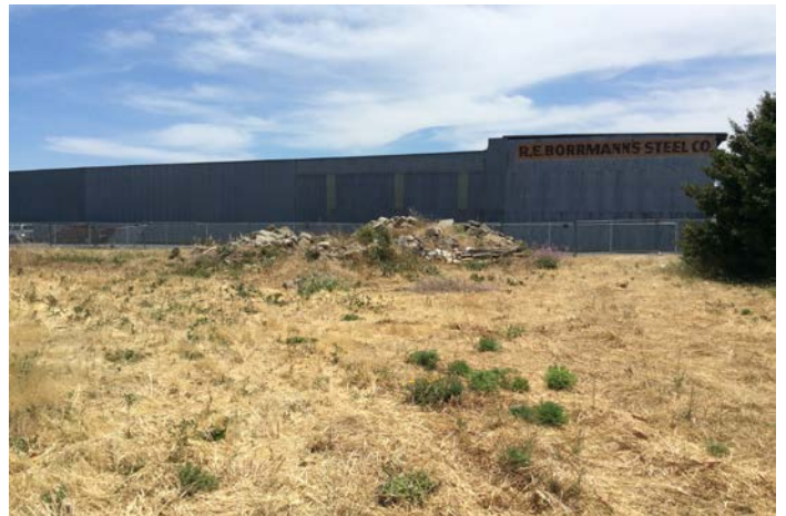
Photo 6: View of debris pile at southern end of site.
