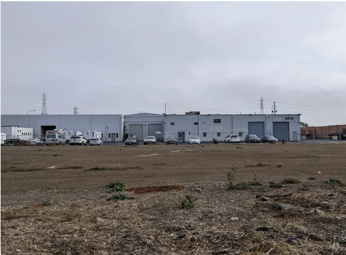
Photo 2: View of the Project Site looking east from the property line.
